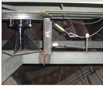
Latch assembly during construction
