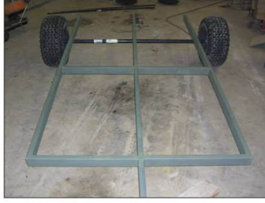
Axle and frame during construction
