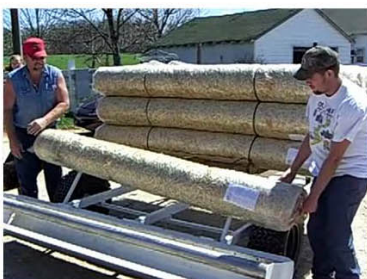
Drop a roll into the dispenser
